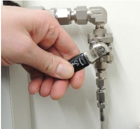
Partly open the Isolation Valve
